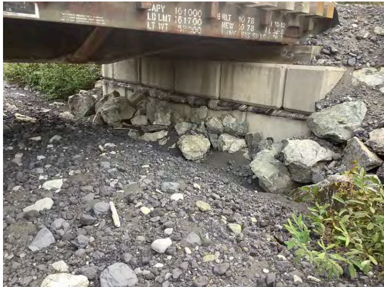
Right Bank Abutment when facing downstream
