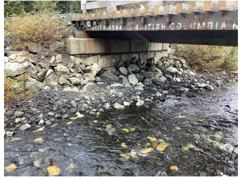
Left Bank Abutment when facing downstream
